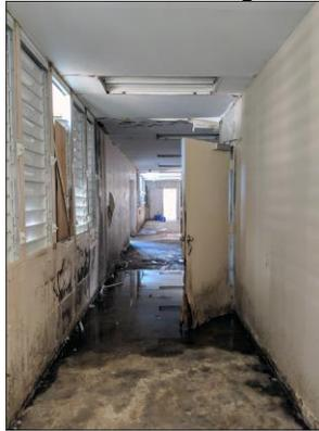
Interior damages to a school in Puerto Rico from water infiltration with standing water and molded walls.
