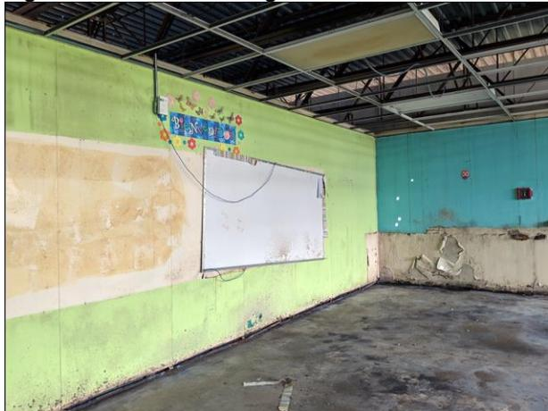
Classroom with mold on floors and water damage on the walls at a school in San Juan, Puerto Rico.
