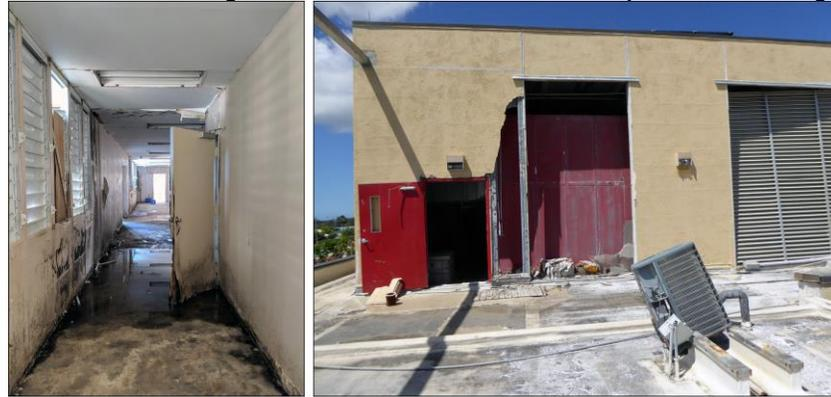
Interior damages to a school in Puerto Rico from water infiltration with standing water and molded walls.
