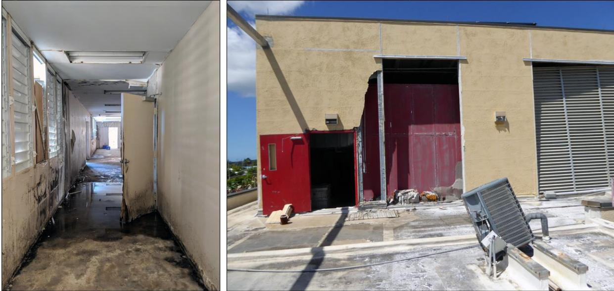
Interior damages to a school in Puerto Rico from water infiltration with standing water and molded walls. Damaged structure and ventilation system at a hospital in St. Croix.
