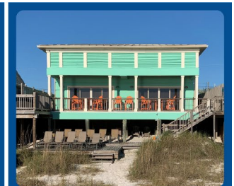
Structure elevation to mitigate flood damage
