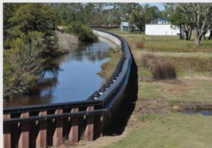
A 5 foot high dike made of steel and concrete built to prevent flooding.
